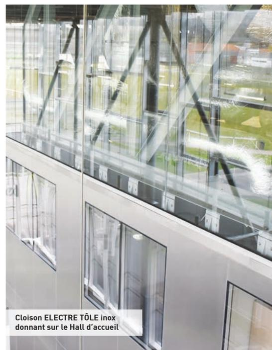
Cloison ELECTRE TÔLE inox
